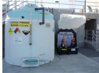
Typical Hydrogen Peroxide Storage Tank and Feed Equipment
